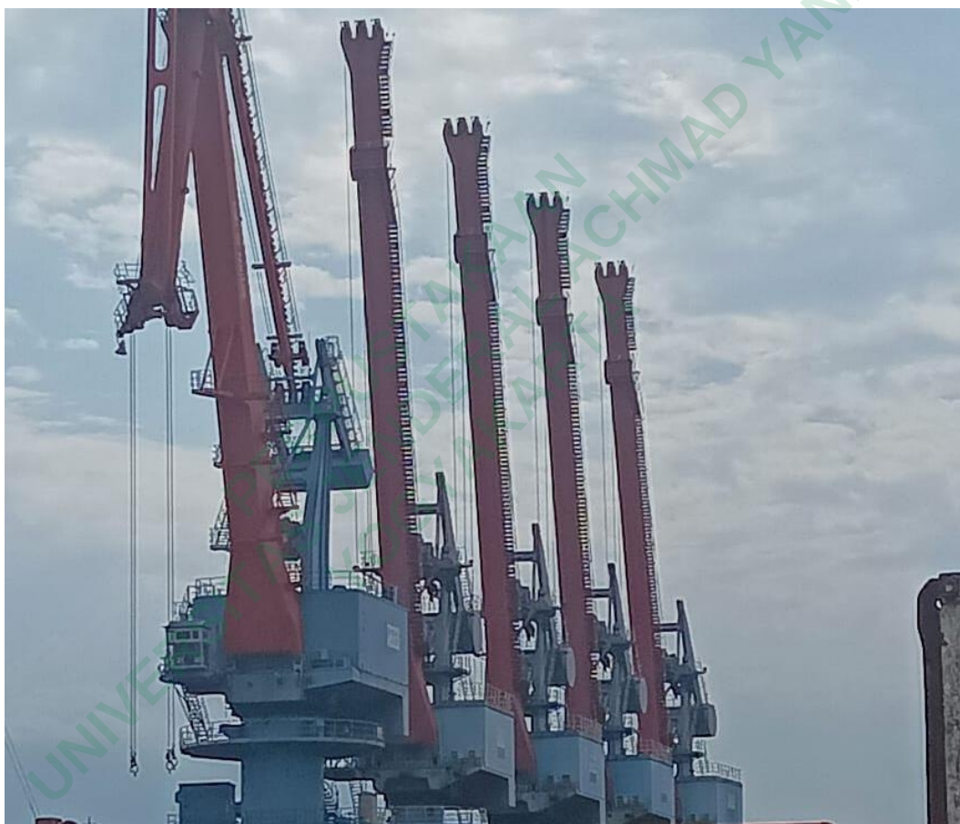
Gambar 3. 1 Gantry Jib Crane
